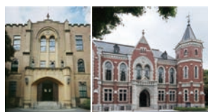
Left: Keio Corporate Administration Building (Jukukan-kyoku) Right: The Old Library [Photo by Ryota Atarashi]
